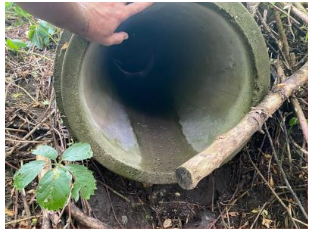
Figure 5: Photograph of discharge pipe onto the Subject Farm
