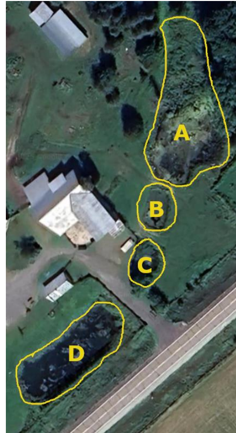
Figure 10: Staged ponds supporting the runoff management system
