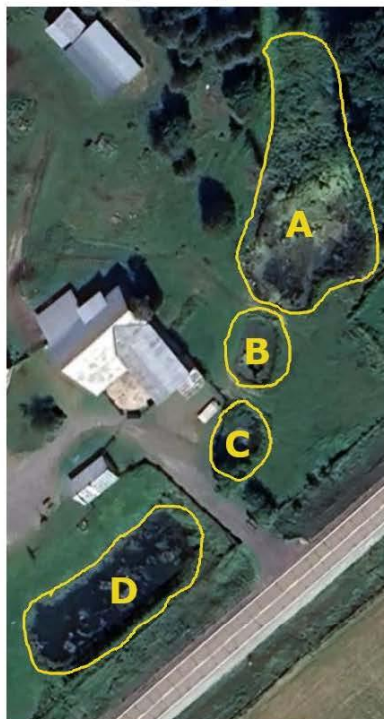
Figure 10: Staged ponds supporting the runoff management system
